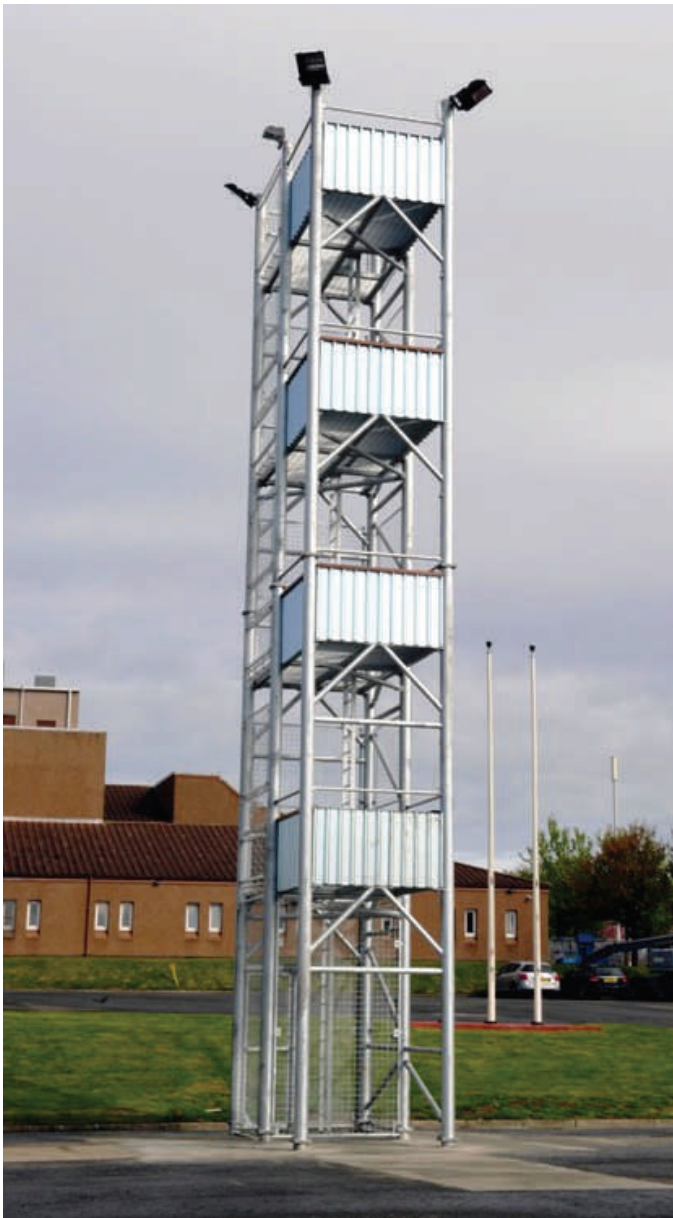
The 1950s training tower (above right) was demolished and replaced with a new steel structure (above).
